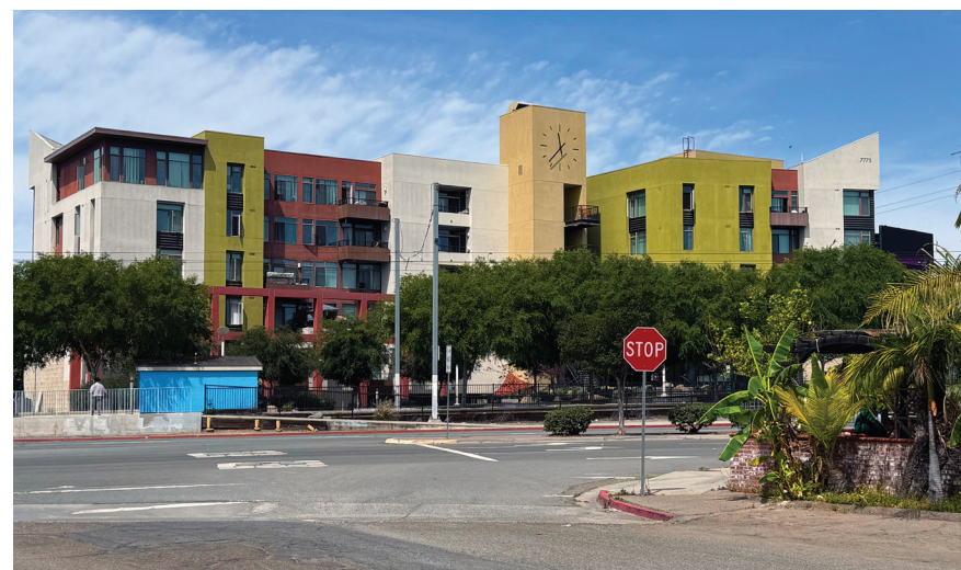
Residential development behind Lemon Grove Depot
