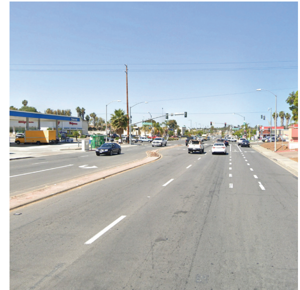
Collector I Street
