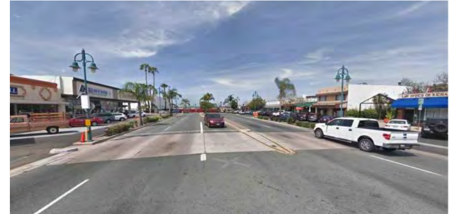
3 RAISED MID-BLOCK CROSSING
