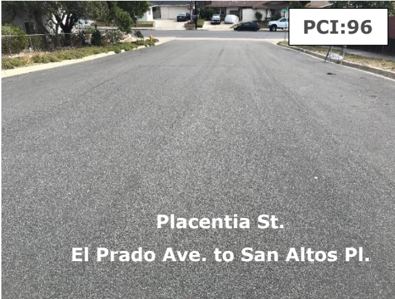
Figure 4. Examples of AC Streets with Different PCIs.
