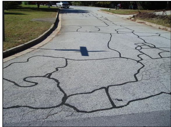
Block Cracking
