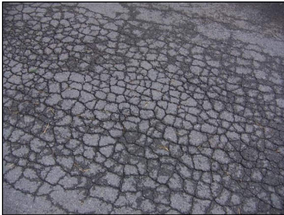
Alligator Cracking
