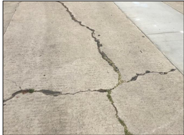
Linear Cracking
