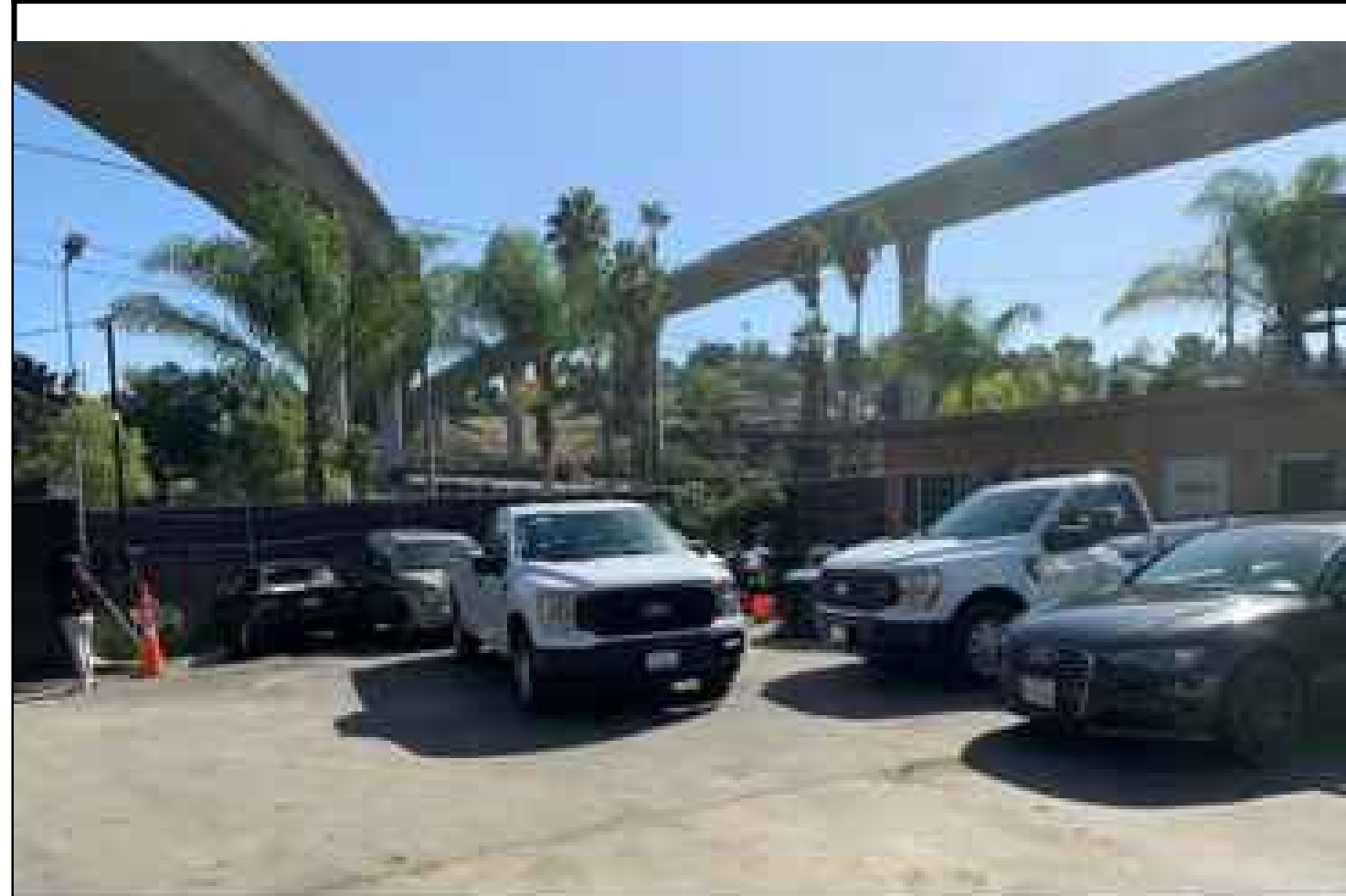
VIEW 24 - SOUTHWEST FAÇADE AND PERIM. AT PARKING
