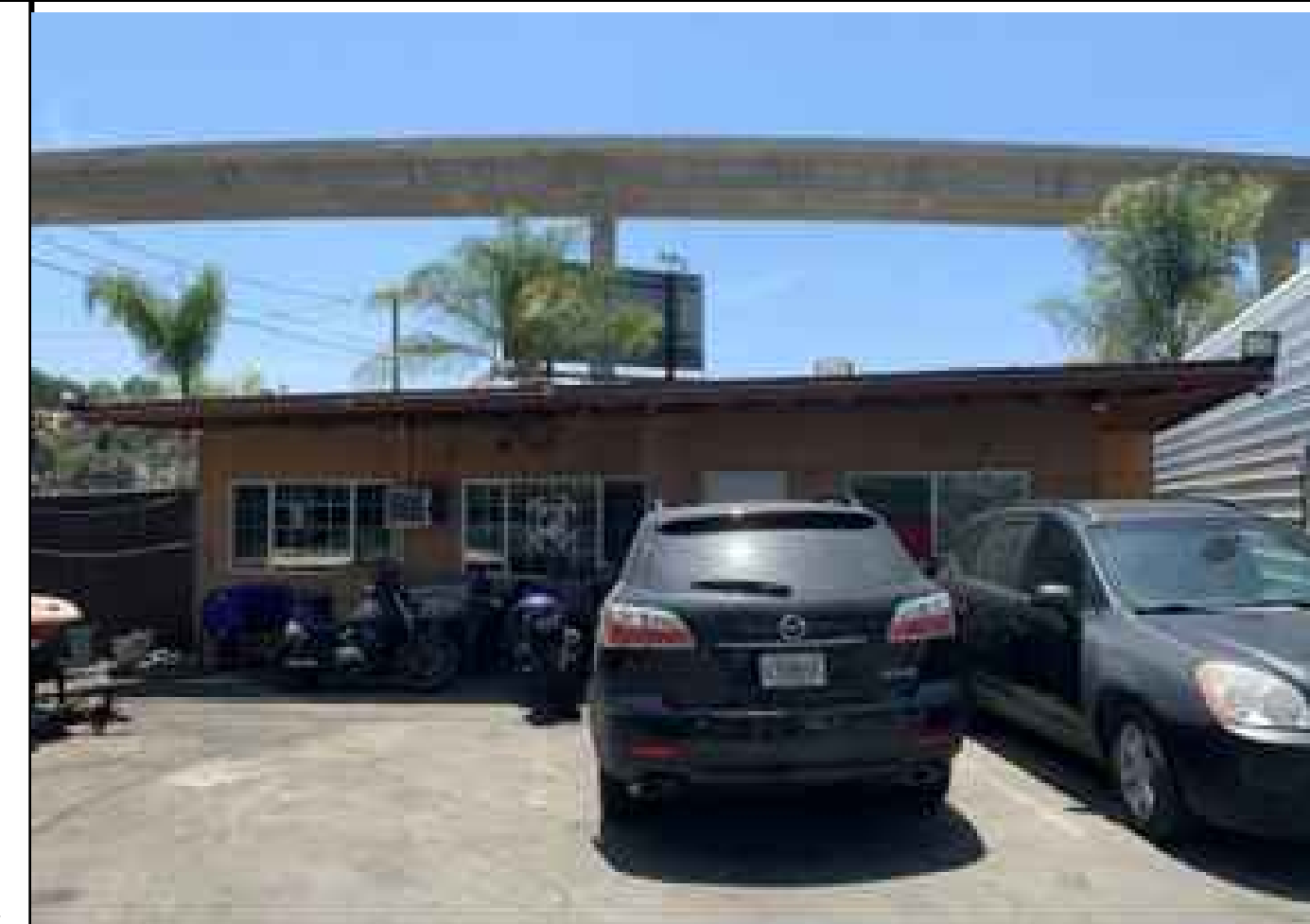
VIEW 9 - SOUTHWEST FAÇADE AT PARKING
