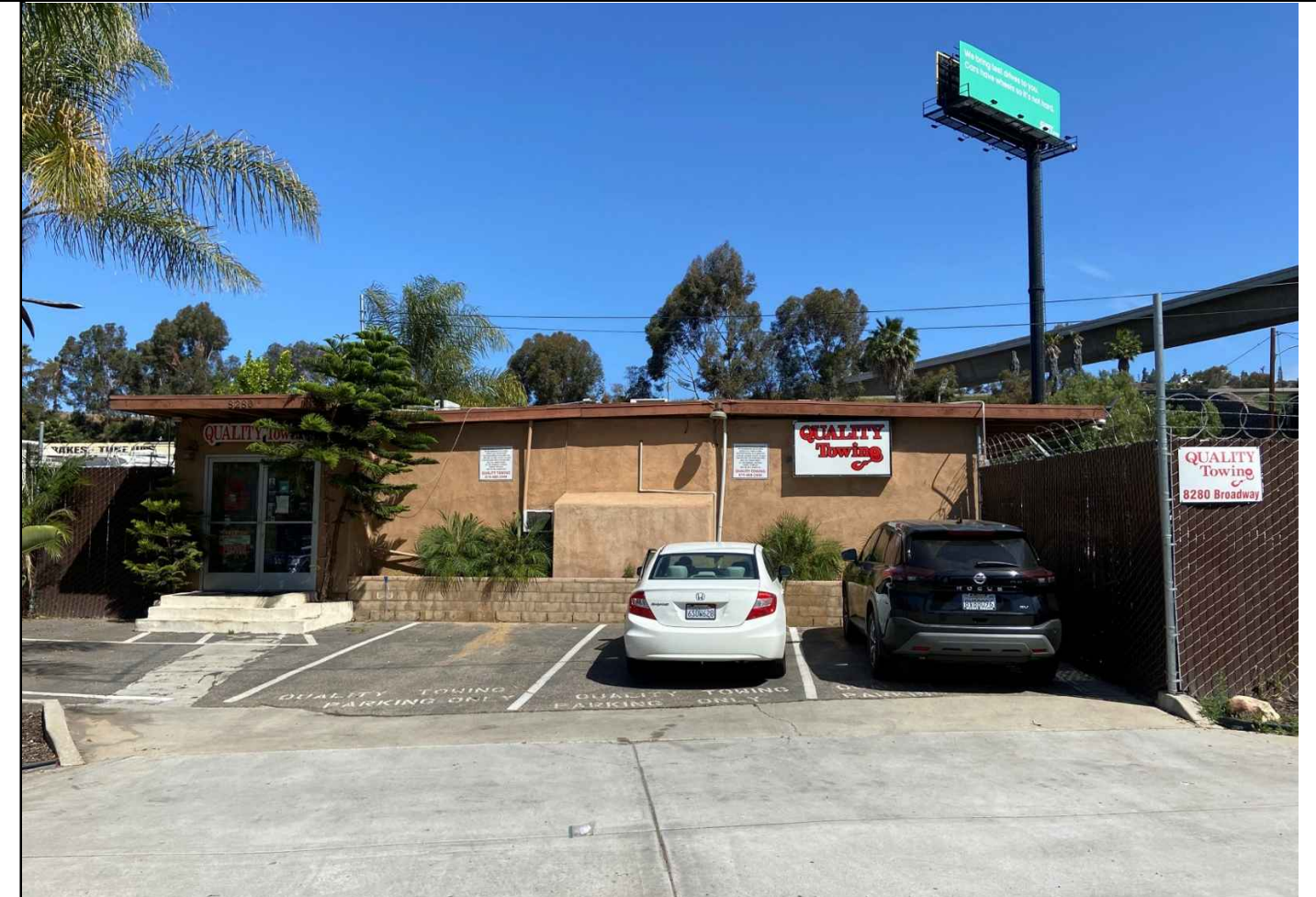
VIEW 6 - NORTHWEST FAÇADE ALONG BROADWAY
