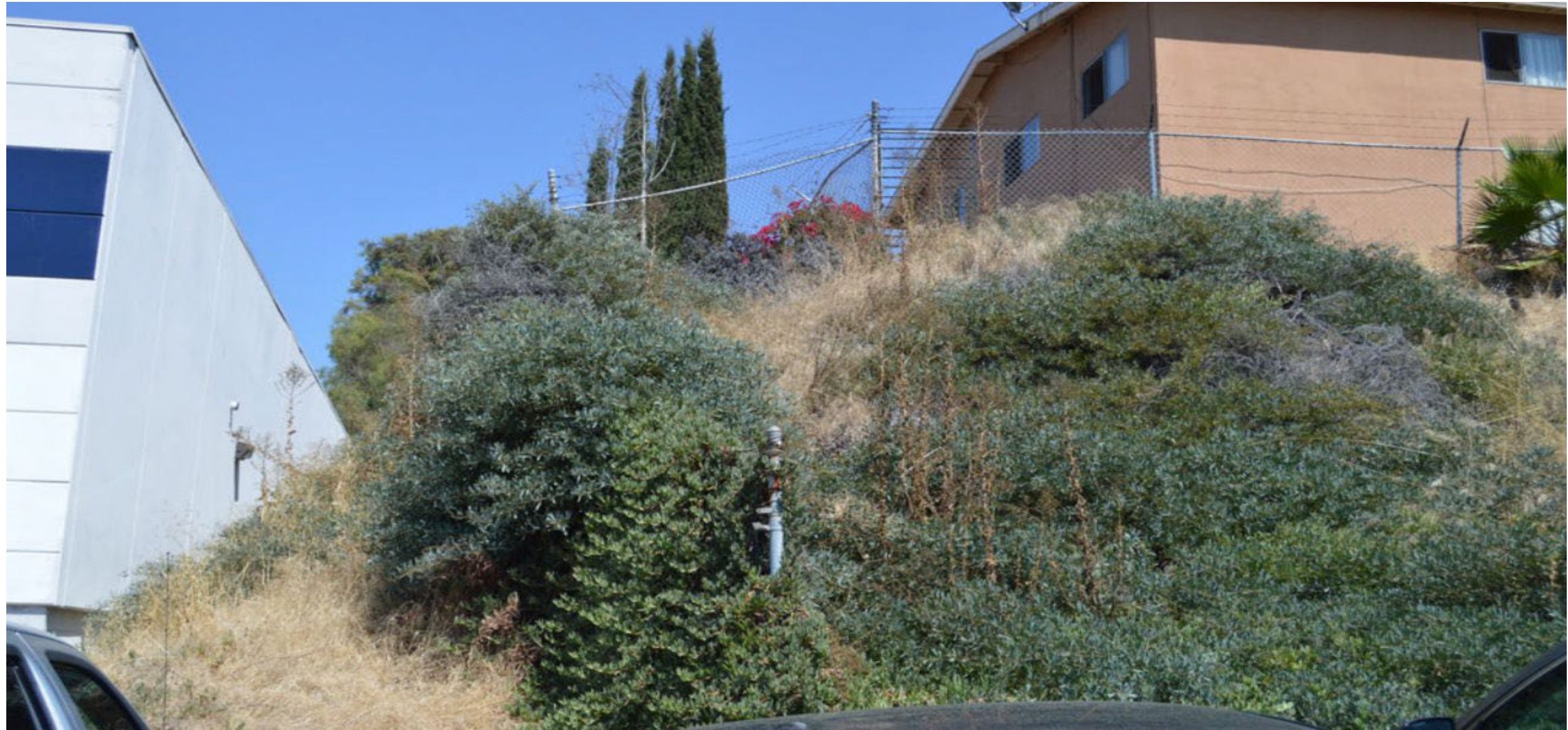
Exhibit 2 -Steep slope of vegetation along the south and east side of the parking lot of the Family Resource Center
