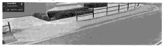
In preparing for this staff report, staff spoke with staff from the City of Poway. Poway has traditionally used DG for a pathway material. However, because DG erodes easily, does not hold up well to heavy foot traffic, and generated frequent calls for repair, Poway began using crushed aggregate base (CAB). CAB is less expensive than DG and has a longer maintenance life. The material is initially rough, but breaks down to a more compact surface over time.
