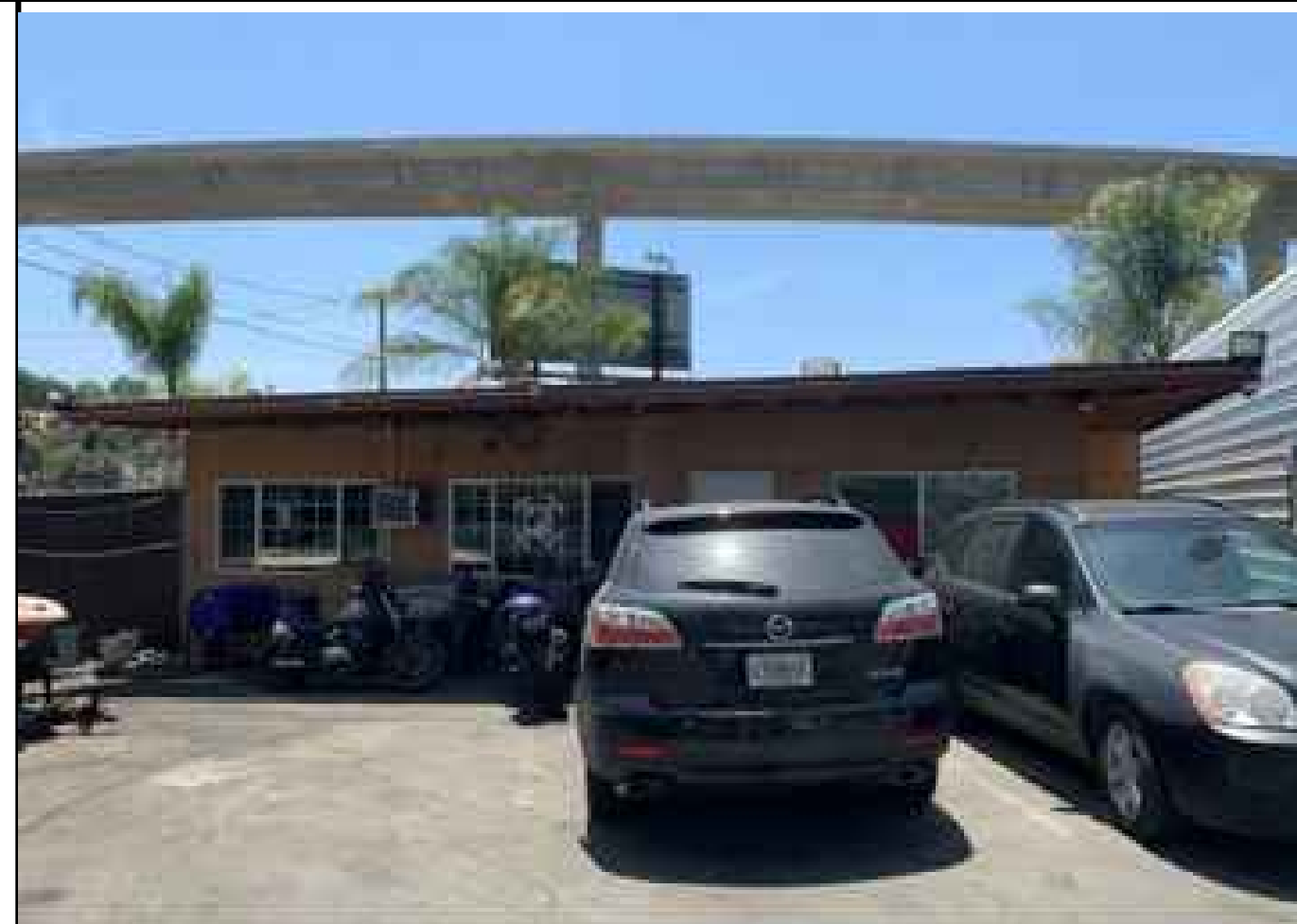
VIEW 9 - SOUTHWEST FAÇADE AT PARKING
