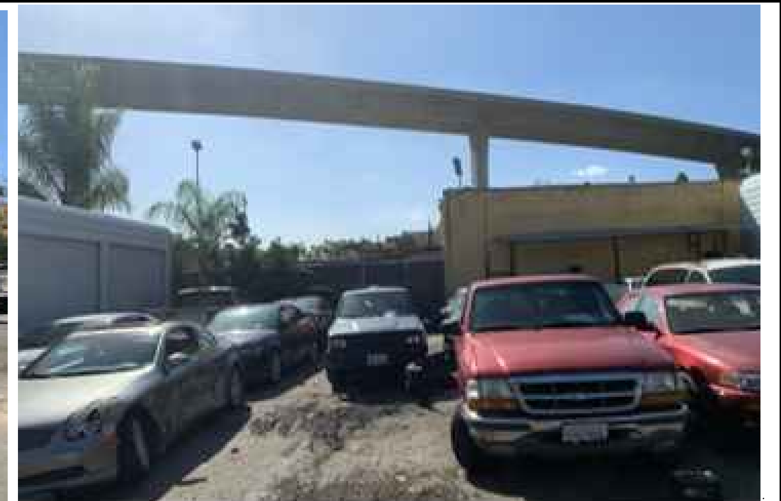
VIEW 11 - SOUTHWEST SHED AT PERIMETER
