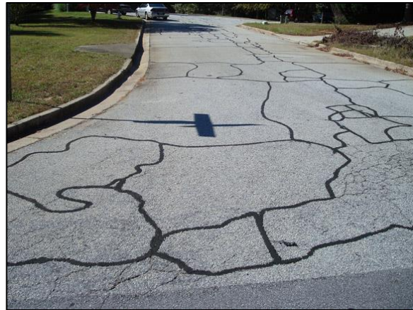
Block Cracking
