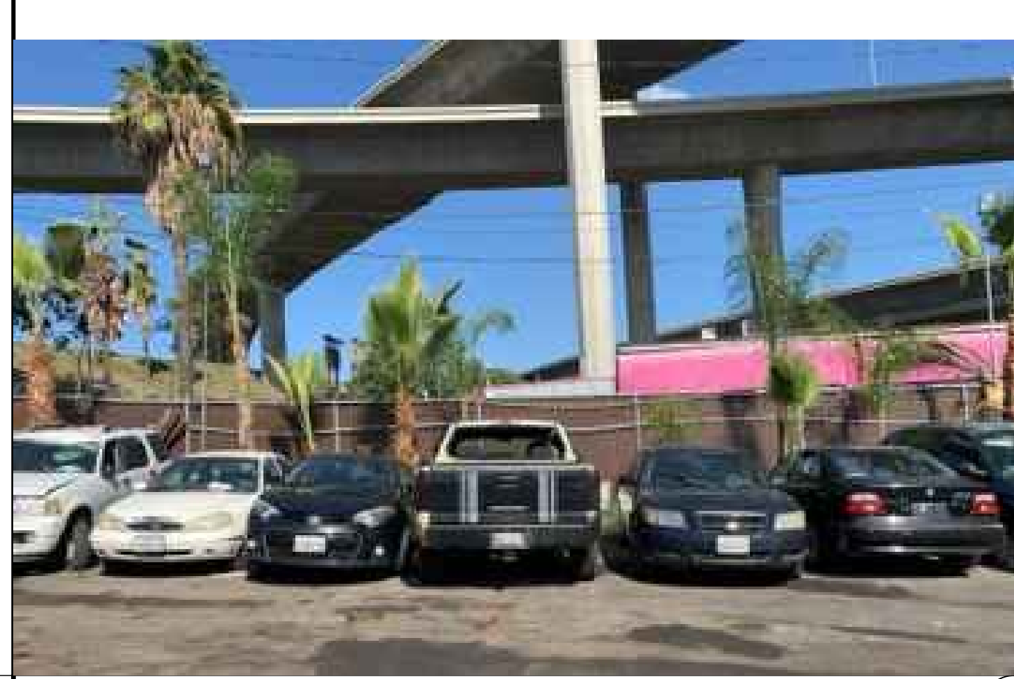
VIEW 19 - NORTHEAST PERIMETER AT PARKING
