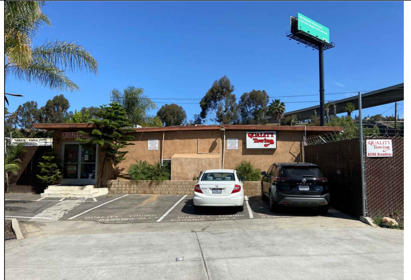
VIEW 6 - NORTHWEST FAÇADE ALONG BROADWAY
